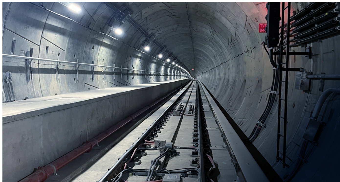
Westside Purple Line Extension Phase 1 (photo courtesy of Los Angeles Metro)
