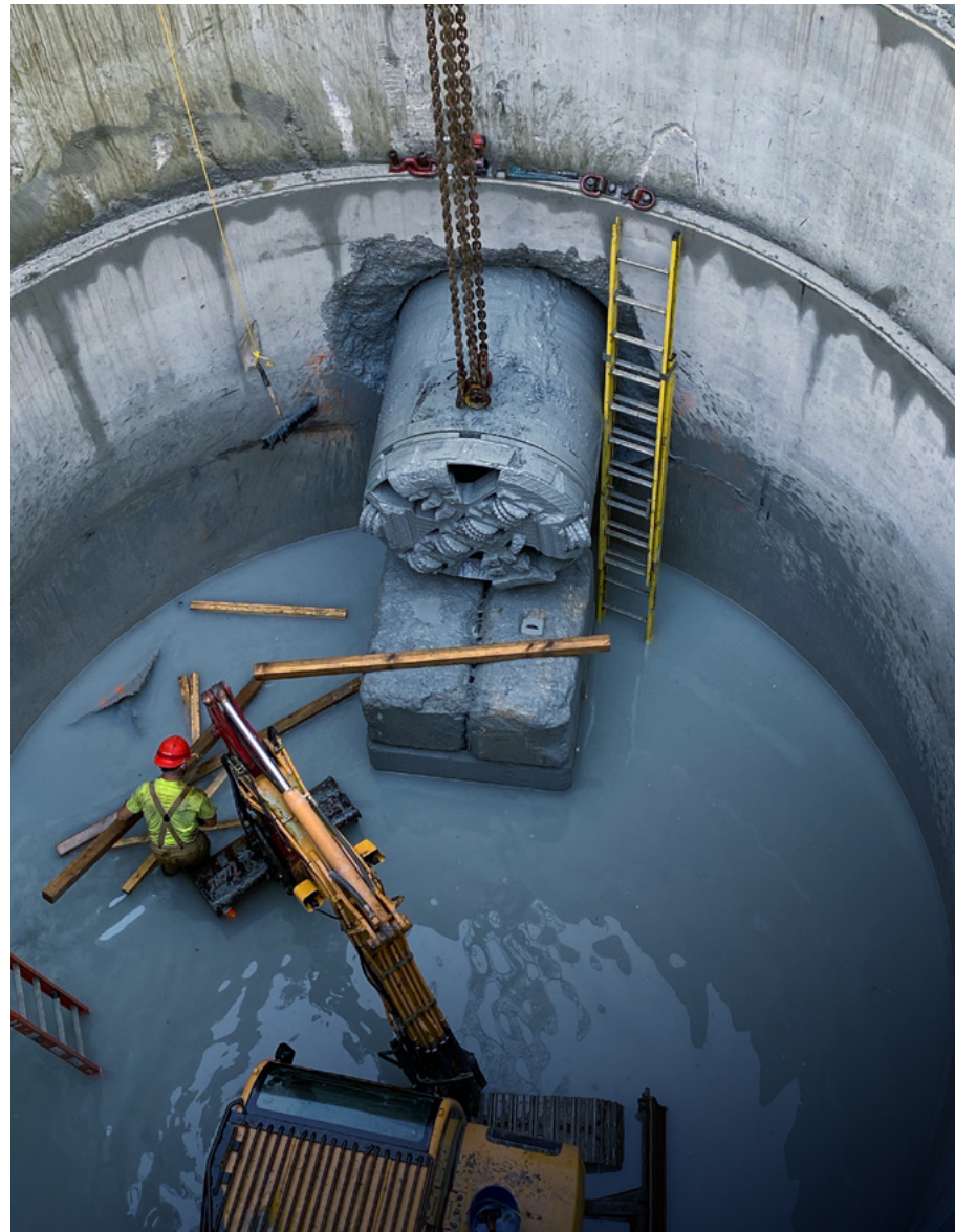
Mattawa Dundas Sanitary Trunk Sewer Project (microtunnel break-out)
