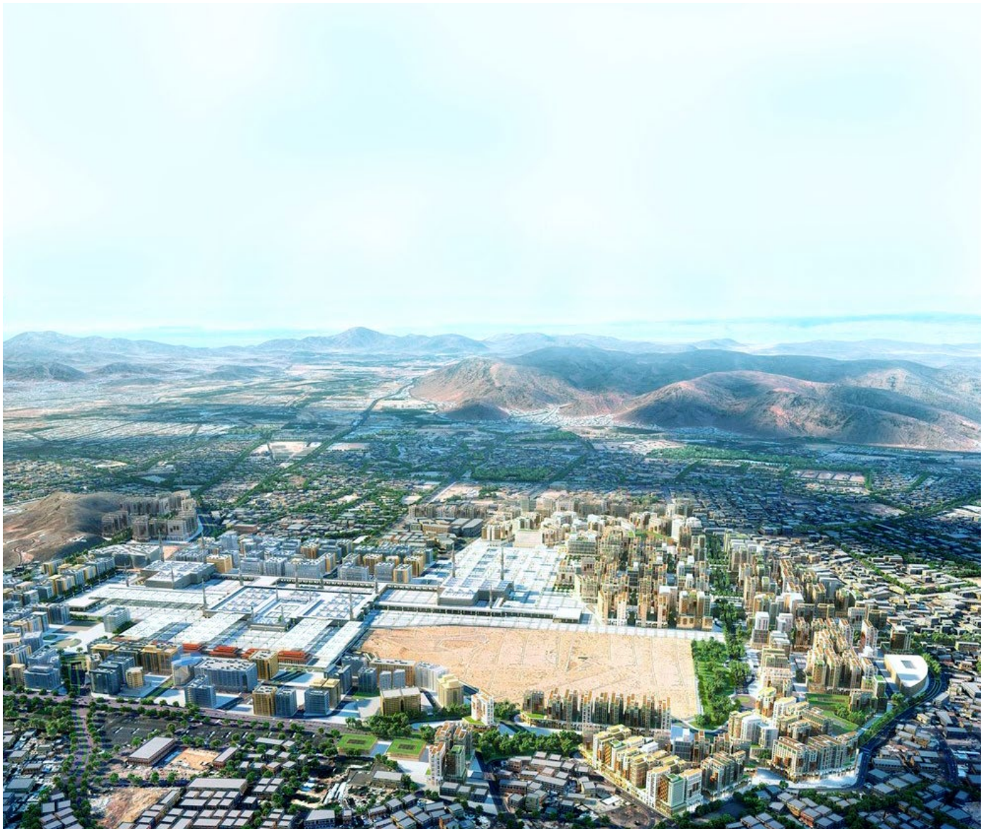
Rua Al-Madinah Project
