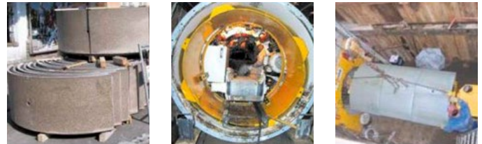
Figure 1. 3-piece 1.3 m dia. polymer concrete segments.
