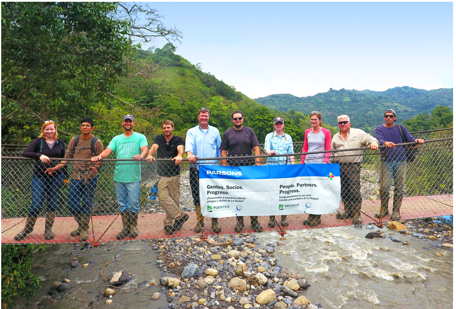
From August 29 to September 6, 2016, a Parsons team—in partnership with Bridges to Prosperity and Puentes de Esperanza—built a new, 58-m footbridge over the La Guaya River in the small village of La Guaya, Colombia (northeast of Bogotá)
