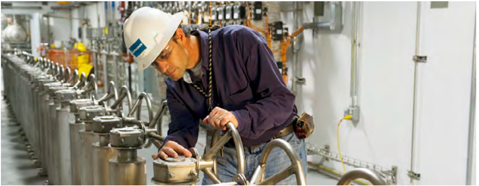
Salt Waste Processing Facility, Aiken, SC
