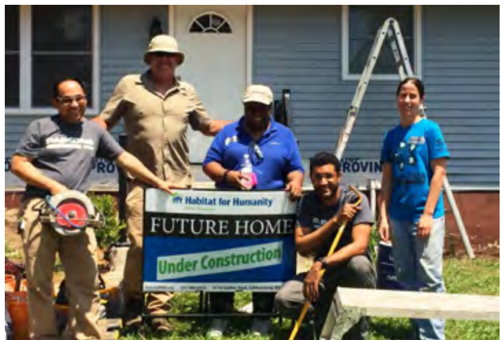
Habitat for Humanity team-building project, Landover, MD
