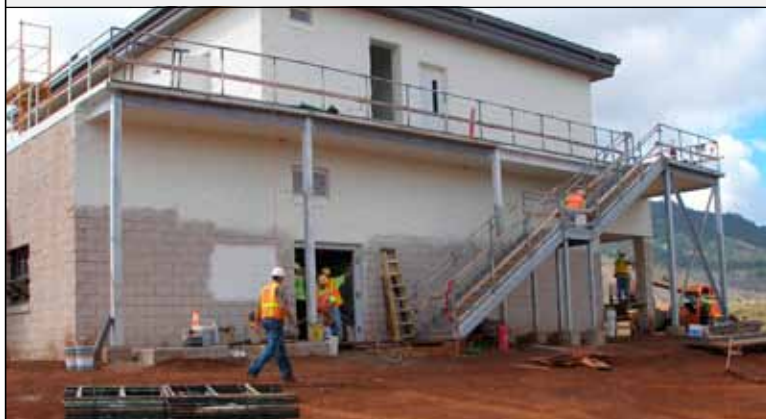
Quarterly construction inspection of Range Operation Center in Hawaii
