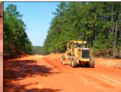
Parsons ITAM crew grading a range road
