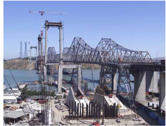
Construction at the new Carquinez Bridge
