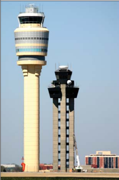
New and existing air traffic control towers
