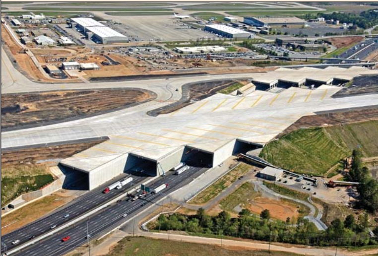
Runway bridge over I-285
