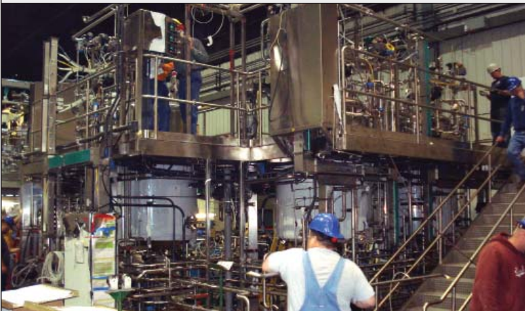
Workers reassemble process equipment in LBXS1 fermentation suite
