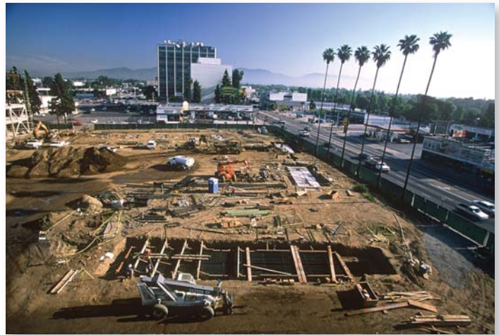
Foundation work underway at a new school in District A.
