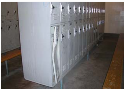
Damaged locker facilities...
