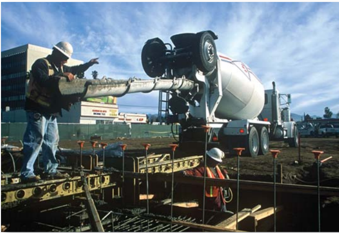
Workers preparing to pour concrete for new construction in District A.
