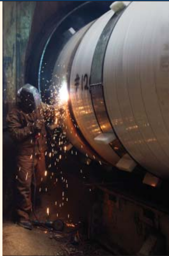
Certified welder joins two pieces of pipe before insertion into tunnel
