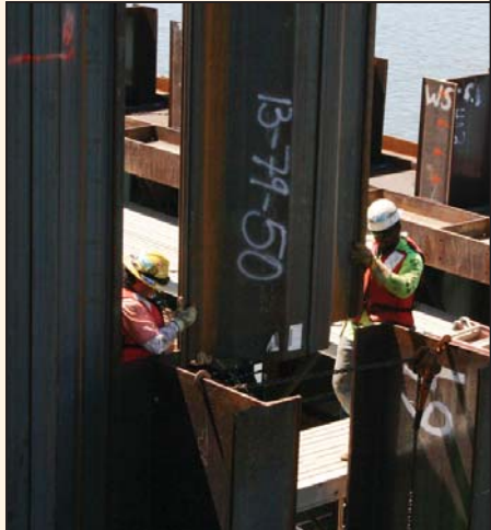
Workers align H-pile to support cofferdam in Sacramento River
