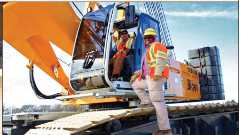
One of several boom cranes operating at intake site
