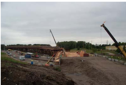
Crosstown bridge near Minneapolis-St. Paul International Airport. This concrete box girder bridge required creative design solutions to satisfy airport air-space requirements.
