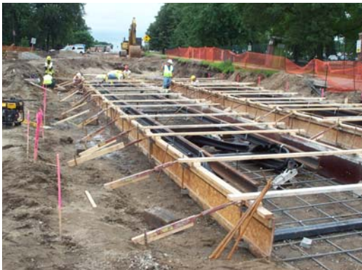
Track construction at Minnehaha Avenue VA Medical Center, South Minneapolis
