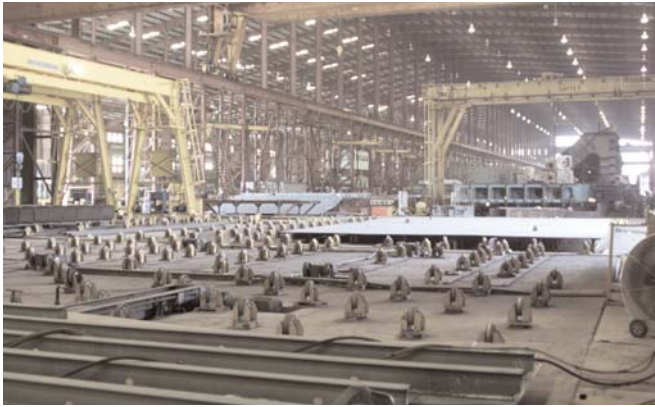
Existing panel shop at Avondale; all new steel fabrication equipment will be installed.
