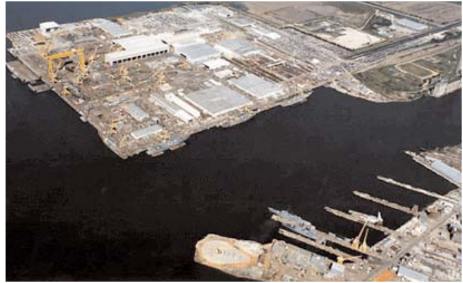
Ingalls operations—the square area above the river was designed and built by Parsons in 1967.
