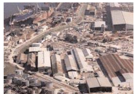
Avondale operations—provides direct access to the Gulf of Mexico via the Mississippi River and the U.S. interstate and rail systems.
