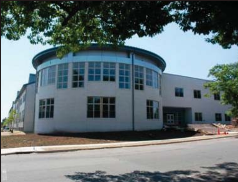
First Avenue District School (side view while under construction)
