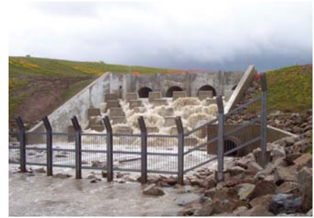
Completed structure in operation during a rain storm.
