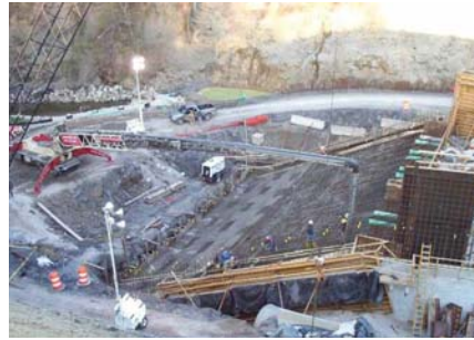
First concrete placement for outlet drop structure.
