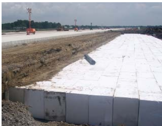
Right: Concrete slabs
