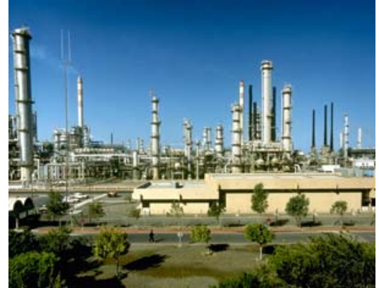
Yanbu's 322,000-bpd Saudi Aramco-Mobil Refinery produces gasoline, diesel, kerosene, fuel oil, and sulfur for export.
